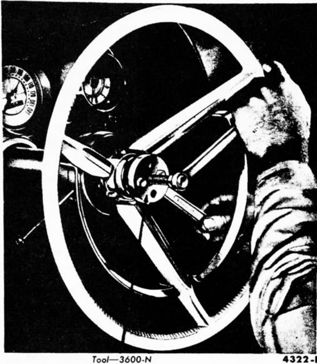
FIG. 4—Steering Wheel Removal
